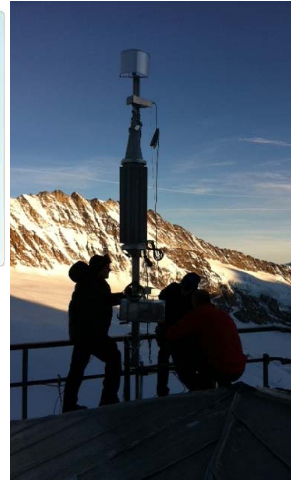
Installation of the new ice selective inlet at the Jungfrauoch
